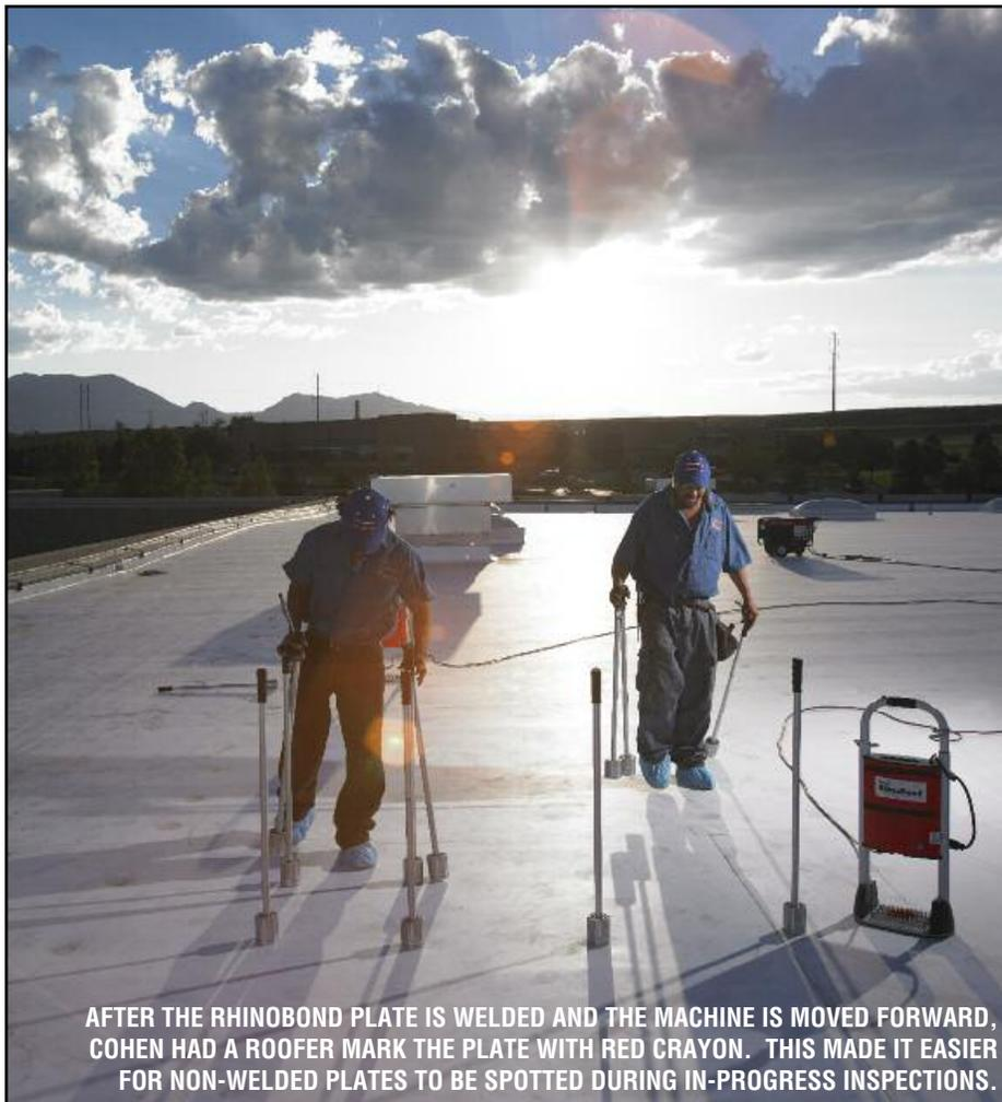
AFTER THE RHINOBOND PLATE IS WELDED AND THE MACHINE IS MOVED FORWARD, COHEN HAD A ROOFER MARK THE PLATE WITH RED CRAYON. THIS MADE IT EASIER FOR NON-WELDED PLATES TO BE SPOTTED DURING IN-PROGRESS INSPECTIONS.
